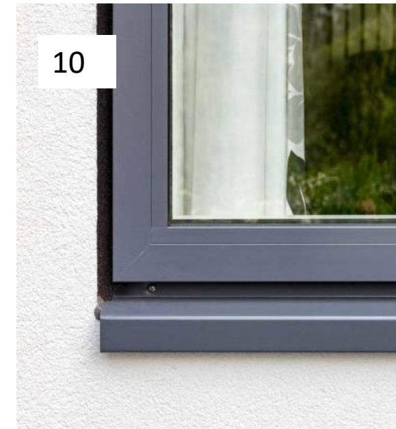
Metal Flashing details
